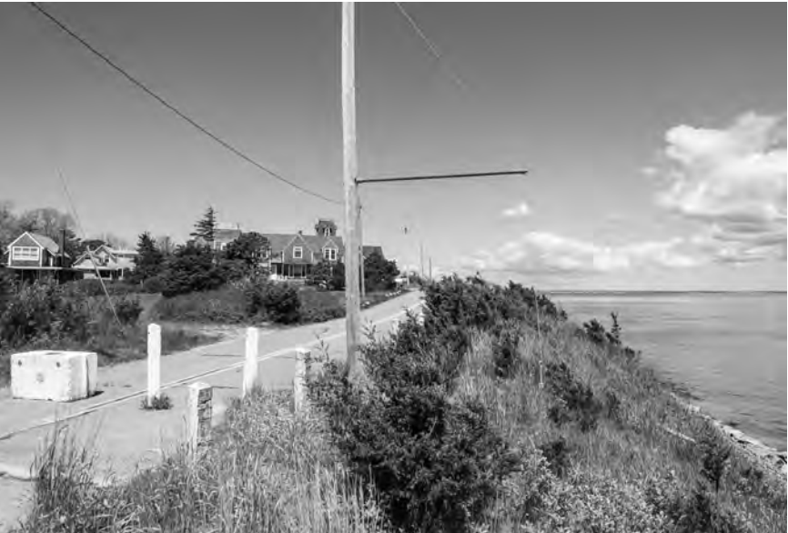
Erosion on the bluffs has long been an issue.
