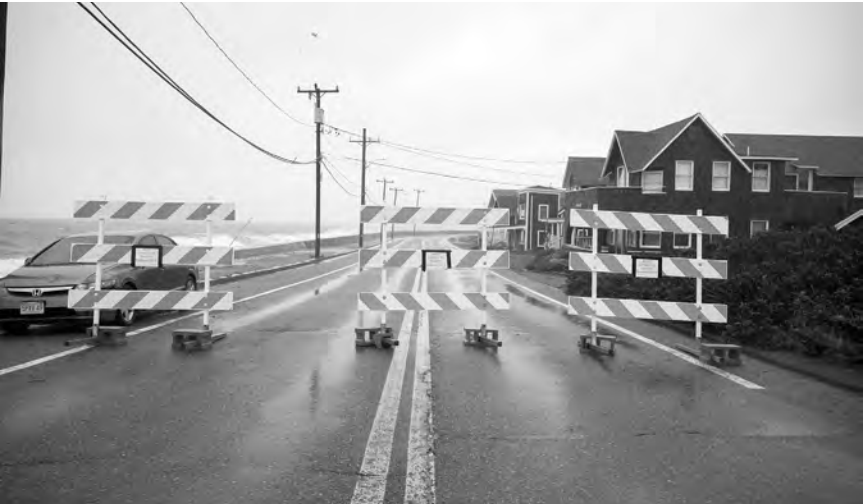
Flooding closed some streets.
